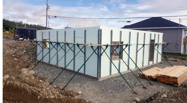
In ICF construction, two insulating faces of a foam block are separated by a connector or web and concrete is poured into the cavity. The foam blocks are left in place to provide insulation throughout the life of the home. Any traditional finish from wood to brick to siding can be applied to interior and exterior faces. On the inside and outside an ICF home can display any architectural style.
